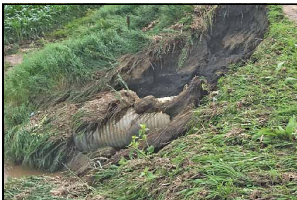
Some of the damages sustained in the recent flooding included large craters and culverts being washed out.
