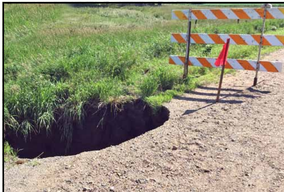
Some of the damages sustained in the recent flooding included large craters and culverts being washed out.
